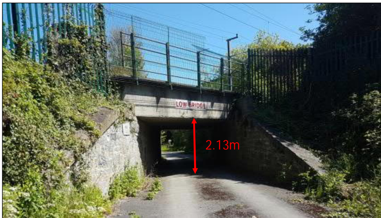
Figure 5.8: Railway bridge underpass on access road
